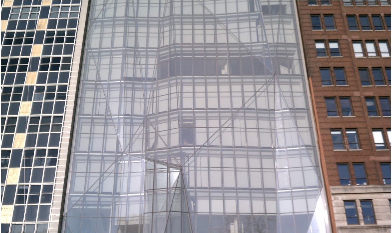
Spertus' glittering facets created by 726 panes of glass in 500 different shapes and sizes is set off against its neighbors. The building is the first LEED museum in the City of Chicago.
